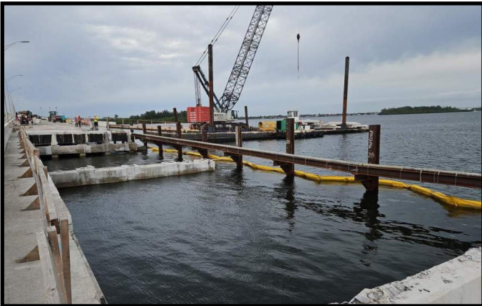
Phase I demolition of deck, barrier wall, and beams.
