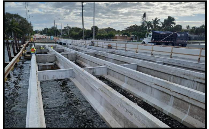
Phase I demolition of deck, barrier wall, and beams.
